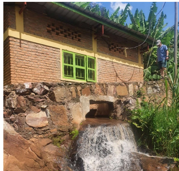
Left: Turbine house and tail-race of pico-hydro project in rural Rwanda
